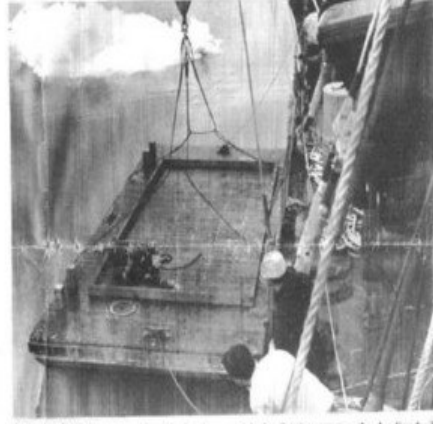
A wooden barge is put over the side. In absence of docks, floating cranes, other landing facilities, it was necessary to discharge convoy's supplies and equipment in two barges like this.
